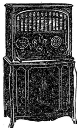
Radiola Super-VIII, an unground Super-Heterodyne. With no outside wiring and no ground connection, it receives far distant stations even while local ones are operating. Loud speaker built in.
