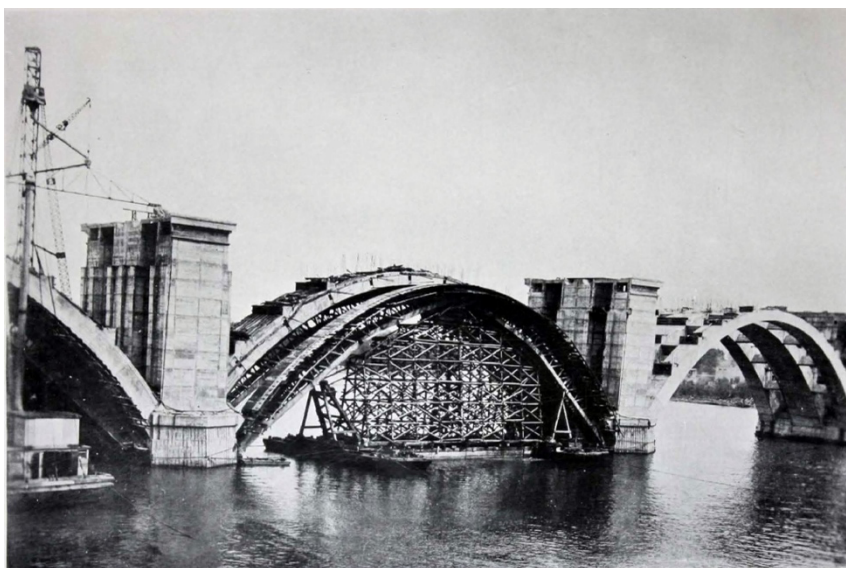
Key Bridge, Georgetown-Washington, D. C. U. S. Engineering Corps. Blaw-Knox steel centering for 208' clear spans being handled with floating equipment using tide to strike and lower centering.
